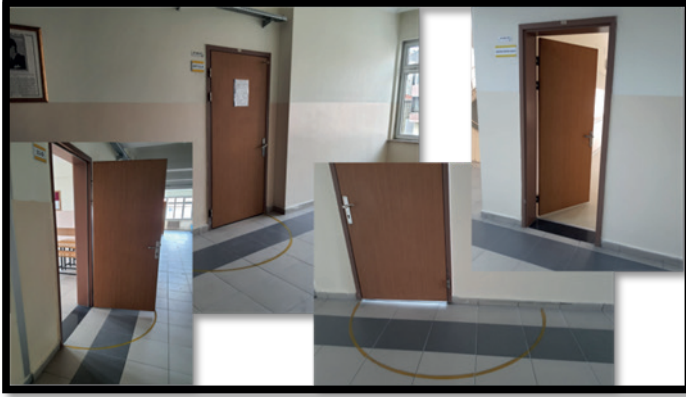
Picture 8: Door Opening Area Lines
