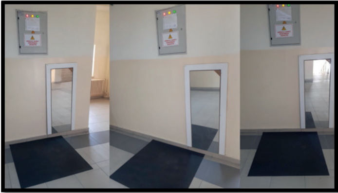
Picture 6: Electrical Panels and Insulator Mats
