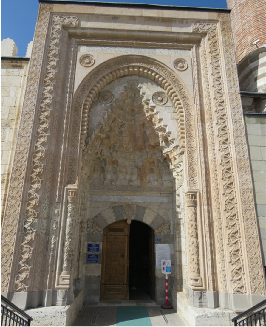
Figure 3: The main portal
