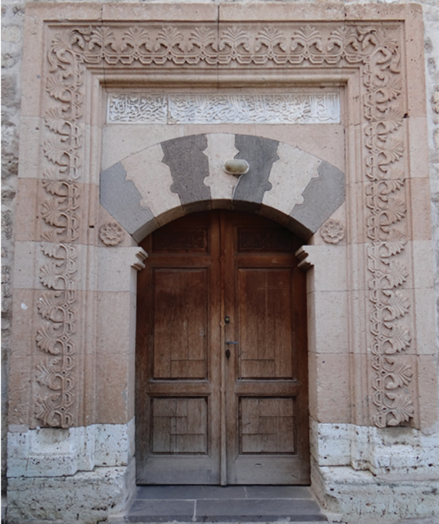
Figure 4: The second portal on the western facade
