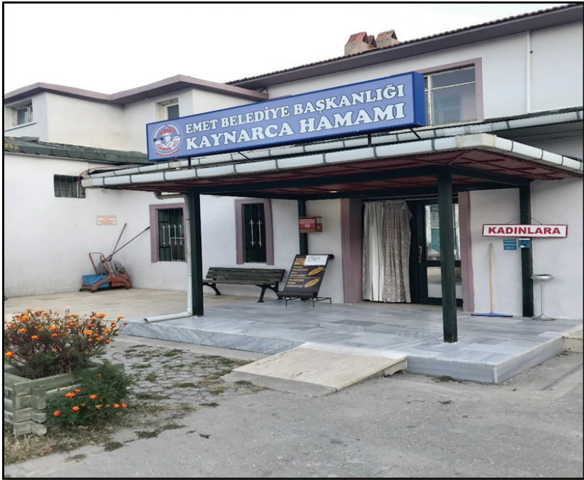
Photo 4. A View from Kaynarca Bath
