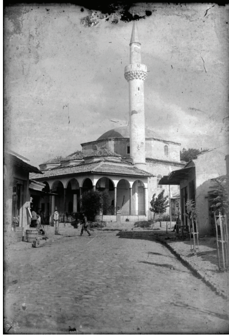
Photo 14- General view from the north-west in the 1940s (Photo. Ahmet Hamdi Yenice) (from Turgutlu City Museum Archive)
