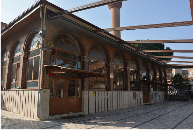
Photo 5-General view from North.
