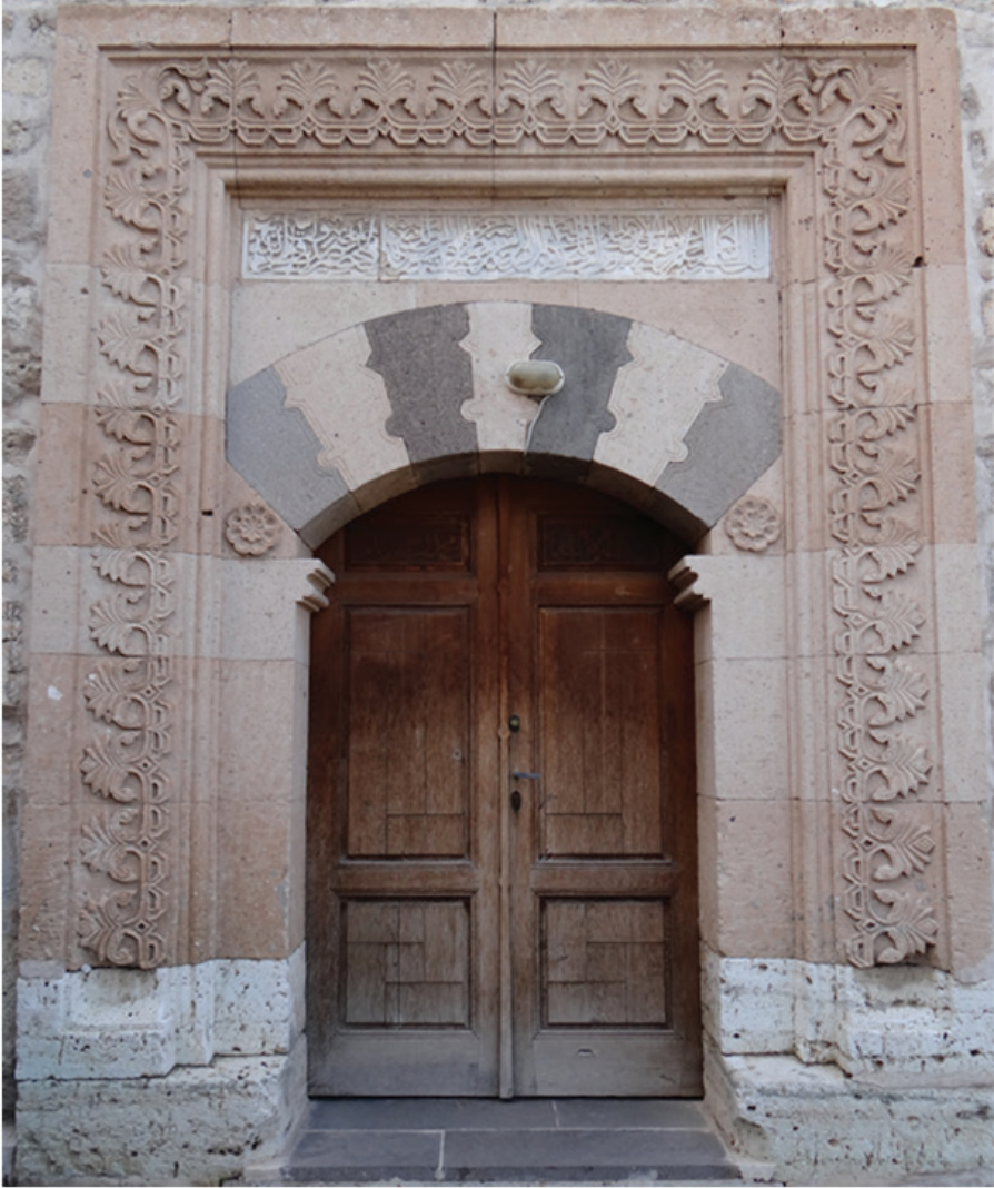
Figure 4: The second portal on the western facade
