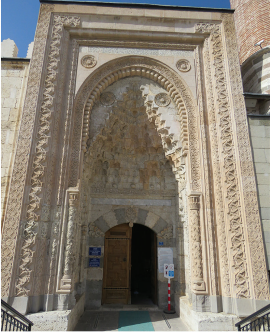
Figure 3: The main portal
