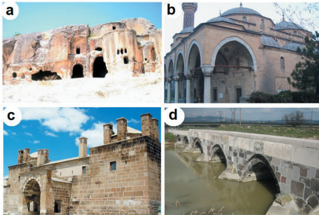
Figure 1. Examples of historical buildings made of tuff and andesite in the Afyonkarahisar region. The Ayazini church was built in the 9th century and is carved inside of a rock mountain, located in the Ayazini district (a), İmaret Mosque was built in 1477, located in the Afyonkarahisar (b), Doger Caravansarie was built in the 15th century, located in the İhsaniye, Afyonkarahisar (c), Altı Göz Bridge was built before 1209, located in the Afyonkarahisar (d).
