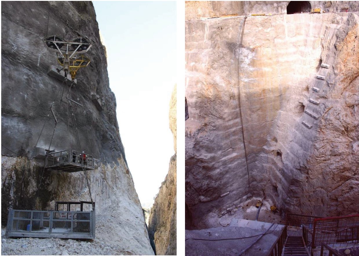
Figure 8. Construction conditions of the prestressed anchors at Ermenek Dam.
