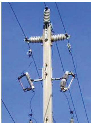
Figure 19. Vibre-type concrete (VBA) pole picture [5]
