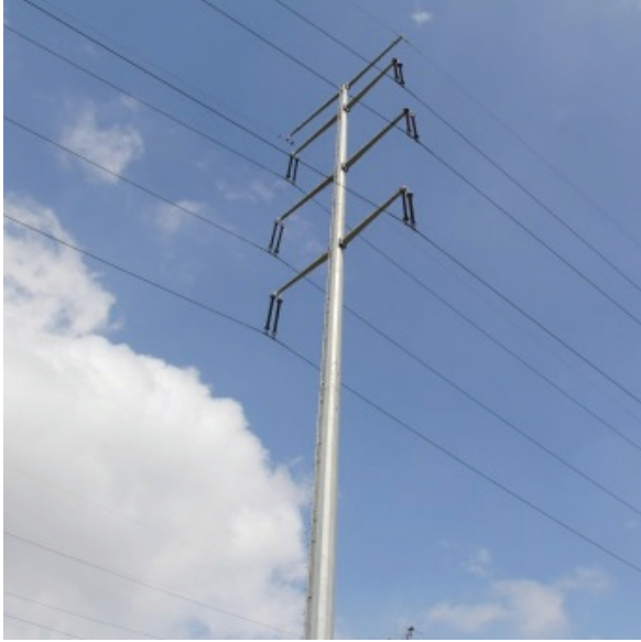
Figure 15. Tubular iron (galvanized) poles [1]
