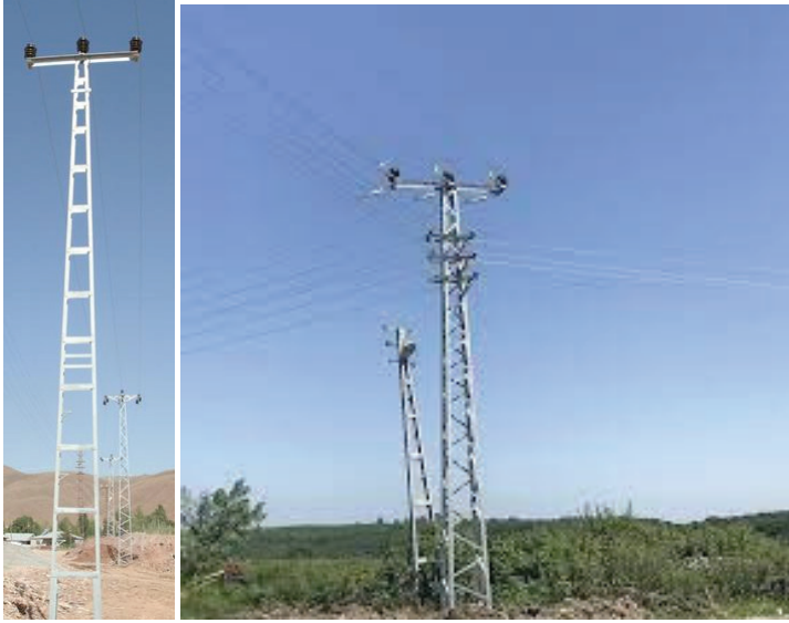
Picture 16. A type and lattice type iron pole pictures
