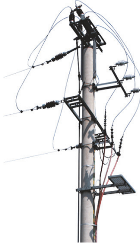
Figure 18. Centrifugal type round (SBA) concrete poles [12]
