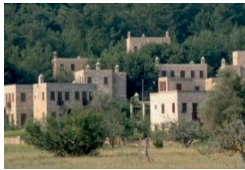
-Scenery, each house placed carefully not to block other ones views
