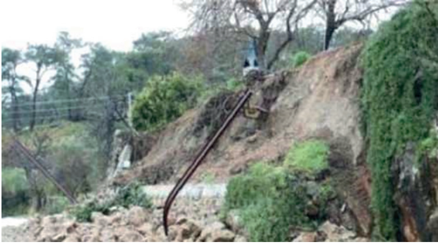
Figure 4. A view of a landslide in Marmaris (Ersoy, 2015).
