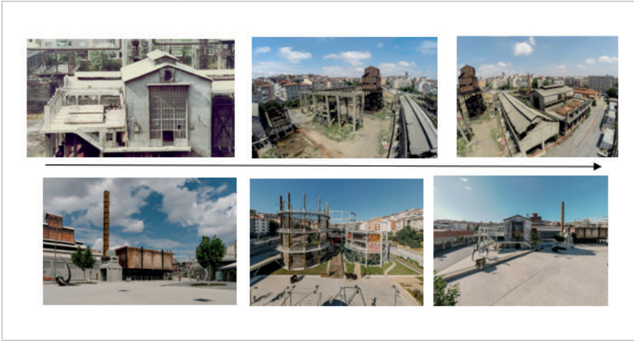
Figure 3 : Hasanpaşa Gasworks → Müze Gazhane
