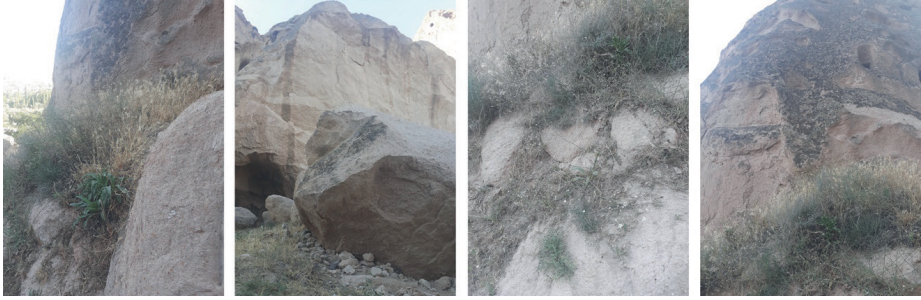
Figure 7. Biological deterioration of Aksaray Selime Cathedral
