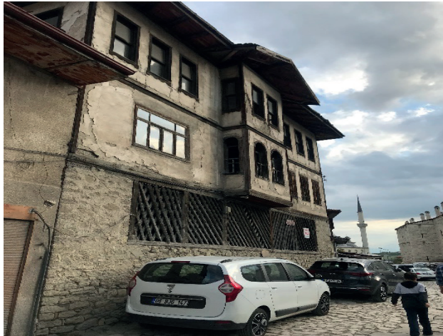
Figure 11. Window that have been altered and expanded in the name of modernization (photo by the author)
