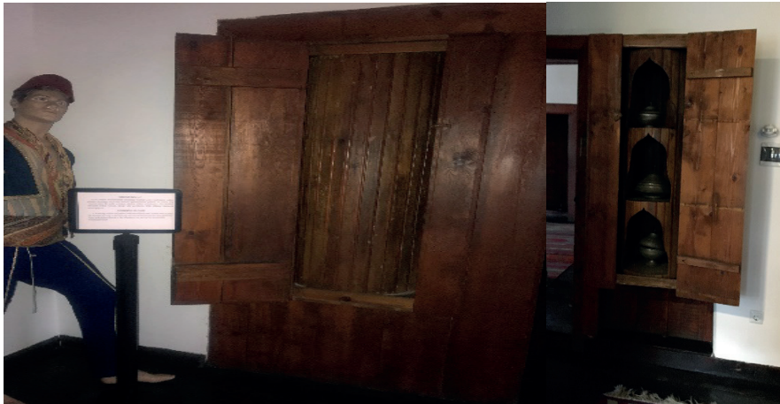
Figure 9. A rotating cupboard (dönme dolap) designed to serve food from the kitchen to the selamlık room (photos by the author from the City Museum).and pillows (photos by the author from Kaymakamlar House Museum)
