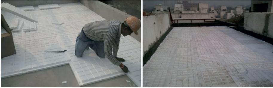
Figure 6. Application images of insulated EPS sheets (Agarwal & Kamal, 2023).
