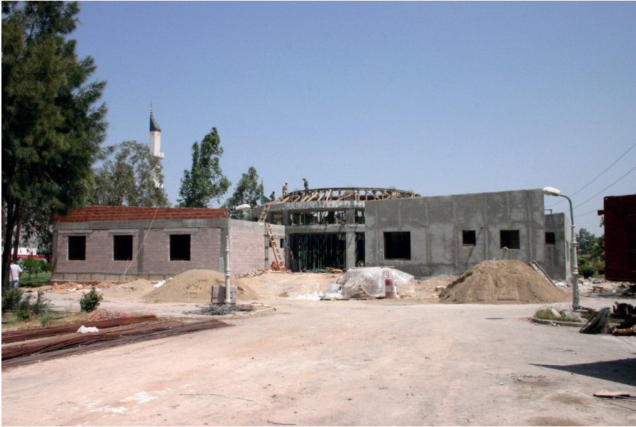
Figure 12. Construction phase (Arno Mimarlık's archive)
