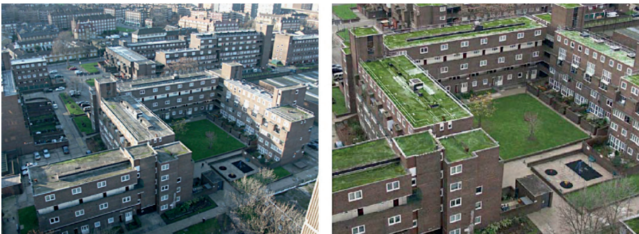
Figure 1. The initial flat roofs at Ethelred Estate were transformed into green sedum roofs as part of the refurbishment process (Castleton et al., 2010).
