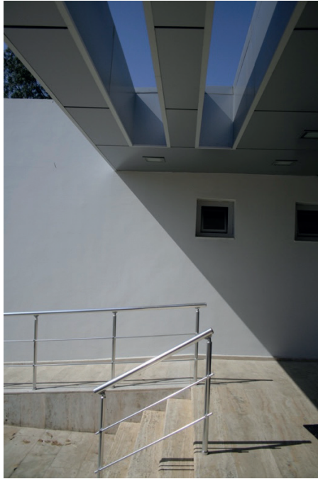
Figure 13. Main entrance (author's archive)
