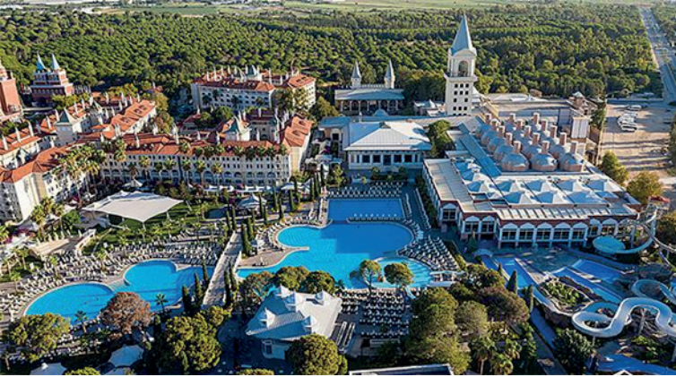
Figure 2: Topkapi Palace Hotel General View
