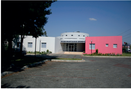
Figure 14. Main Facade of the building (author's archive)
