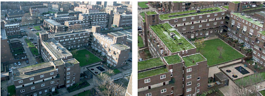
Figure 1. The initial flat roofs at Ethelred Estate were transformed into green sedum roofs as part of the refurbishment process (Castleton et al., 2010).
