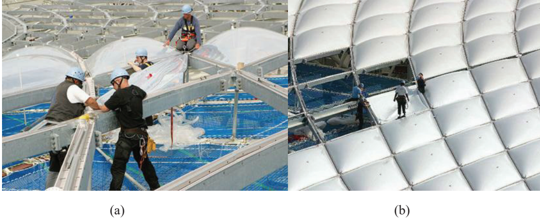
Figure 21-(a,b) Installation of ETFE cushions in their places (URL-22, URL-19)
