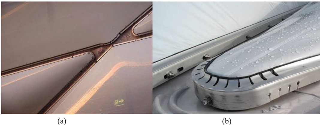
Figure 23-(a) spring-loaded steel plate bed (URL-22) that will move with expansion, (b) spring-loaded steel plate (URL-22)
