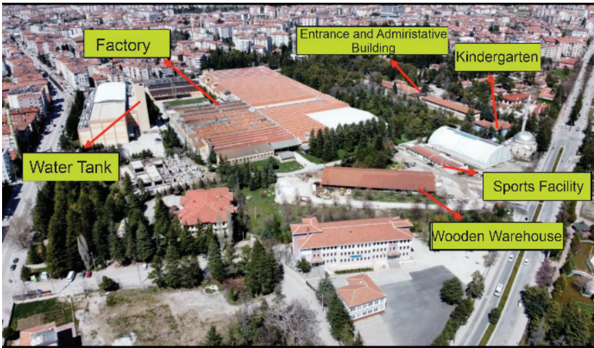
Figure 5. Weaving factory and nearby buildings (Kocadağ, 2022)
