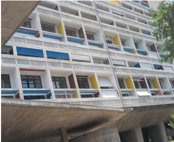
Fig. 8. Unite d'Habitation Marseille, Le Corbusier The raised columns called pilotis Photo, H. Coskun, 2011.
