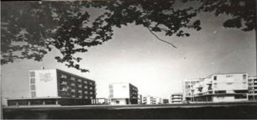
Fig. 10. Istanbul, Levent project, after Henri Prost re-planned by K.A. Aru, R. gorbou. Photo, A.Avcı.
