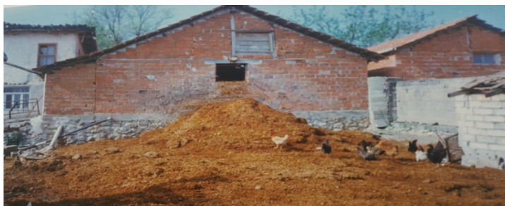
Figure 10. Manure discharge opening in a barn
